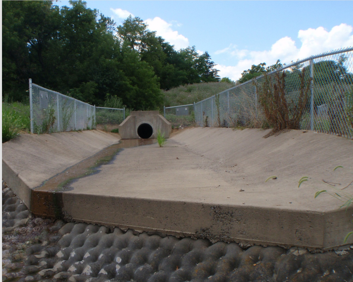
Flow at University Park due to a broken water line
